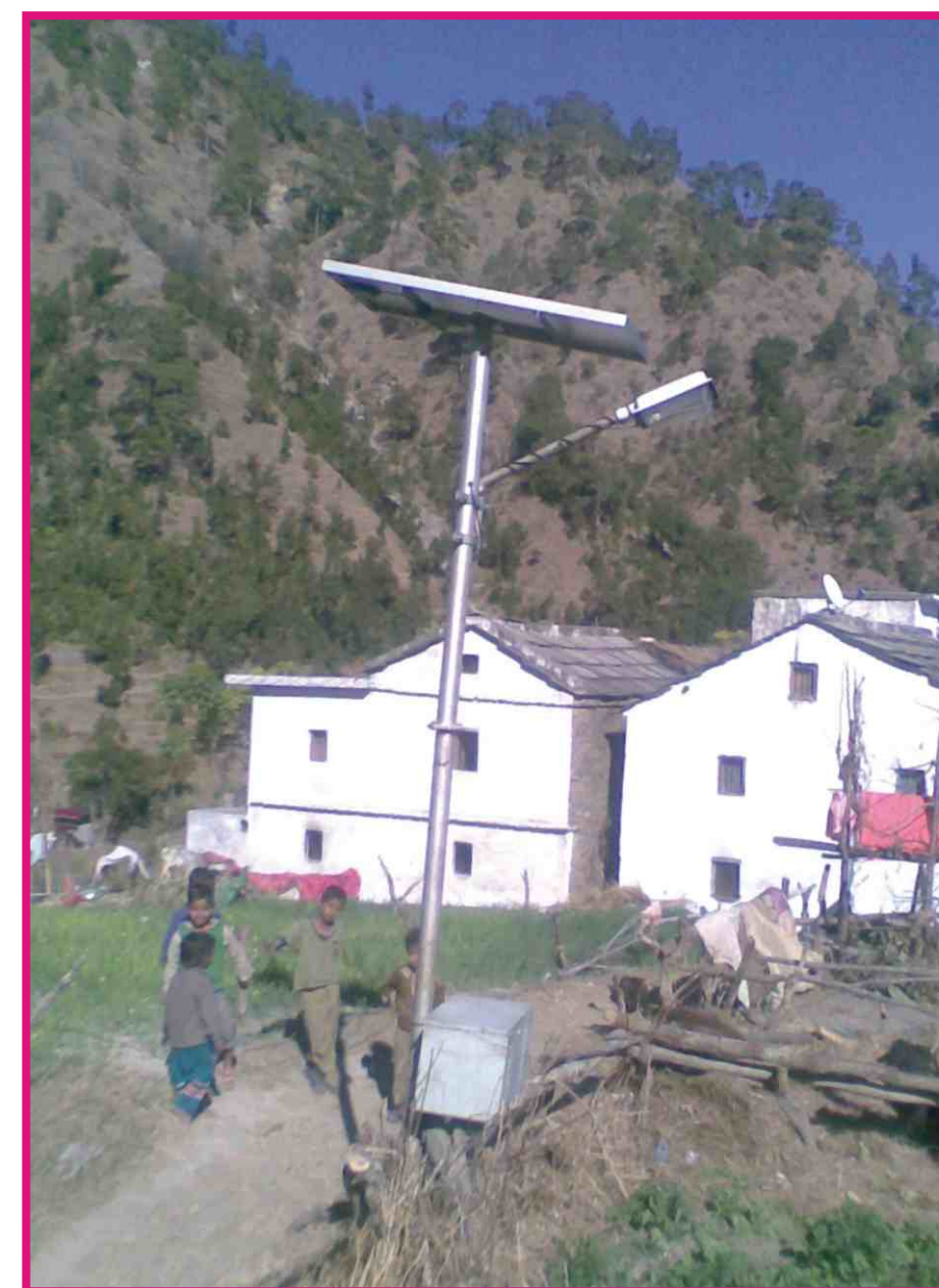
Solar Street Light in Unelecteified Remote Area
